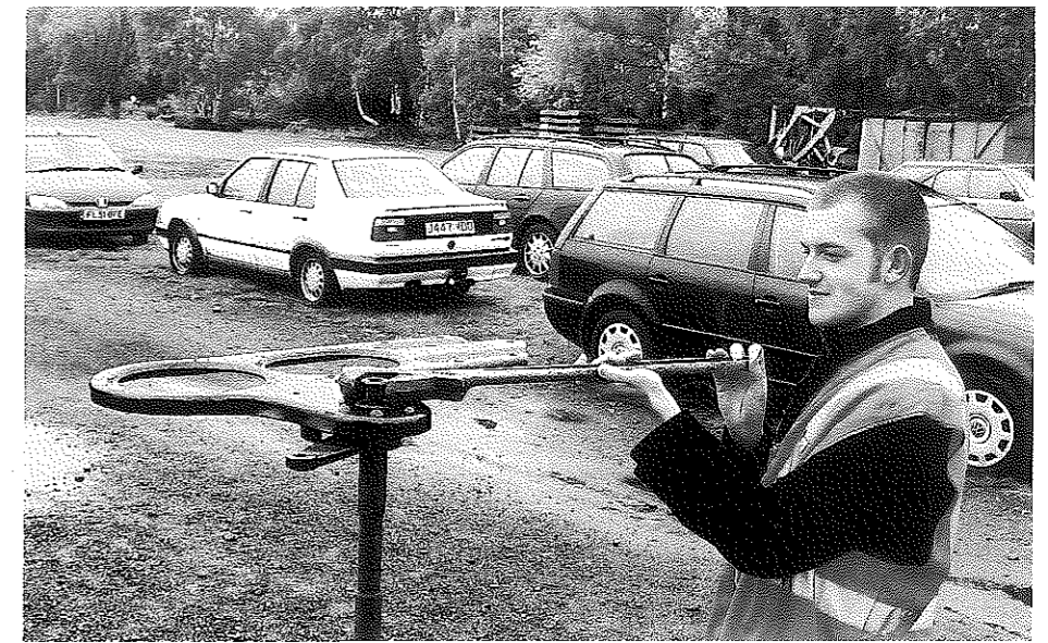
Adding the spindle casting to the spectacle plate for a signal arm, using the longest spanner I've ever seen! RICHARD NAPIER.
